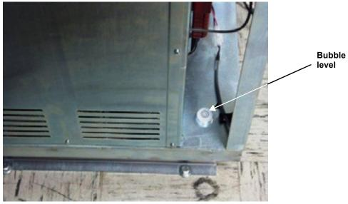
13. Once the cabinet is level, firmly tighten the front bolts to drop-in anchors as shown in **Figure 134**. The front bolts must be tightened to 40 foot-pounds (54 N-m) of torque.
